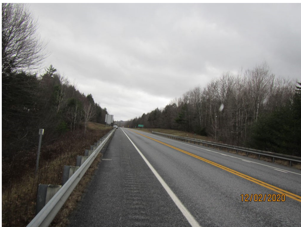
Picture 2: Looking south on US Route 7 over Bridge 19-7
