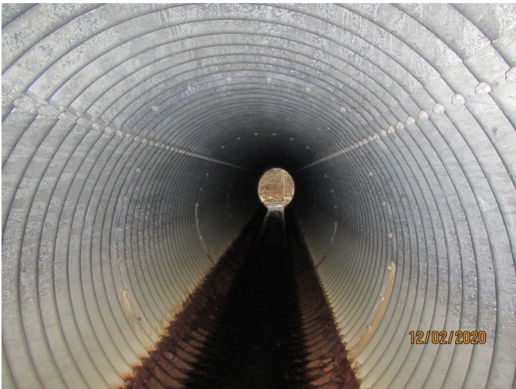
Picture 6: Culvert Barrel
