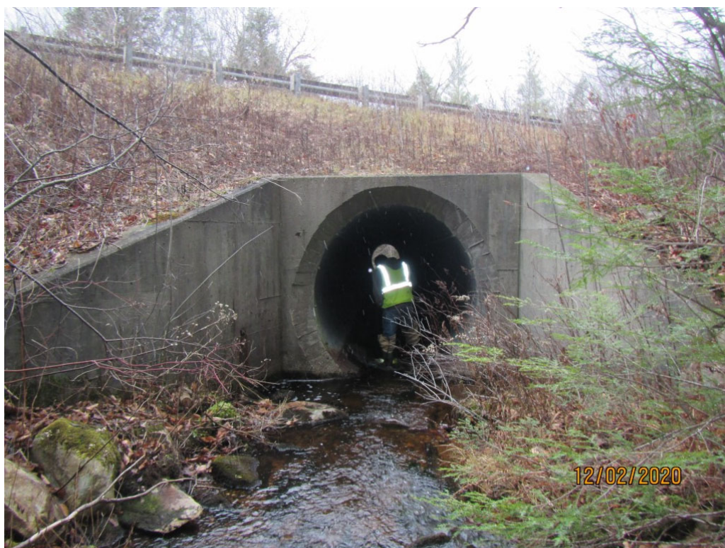
Picture 4: Bridge 19-7 inlet
