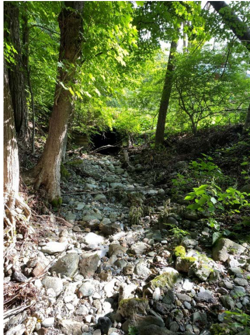
Photo 15. Photo view looking north towards the inlet of BR 61 where it crosses VT-30. Photo view shows culvert dry streambed conditions and some evidence of dynamic channel with exposed roots on mature trees. Stantec, July 19, 2022.
