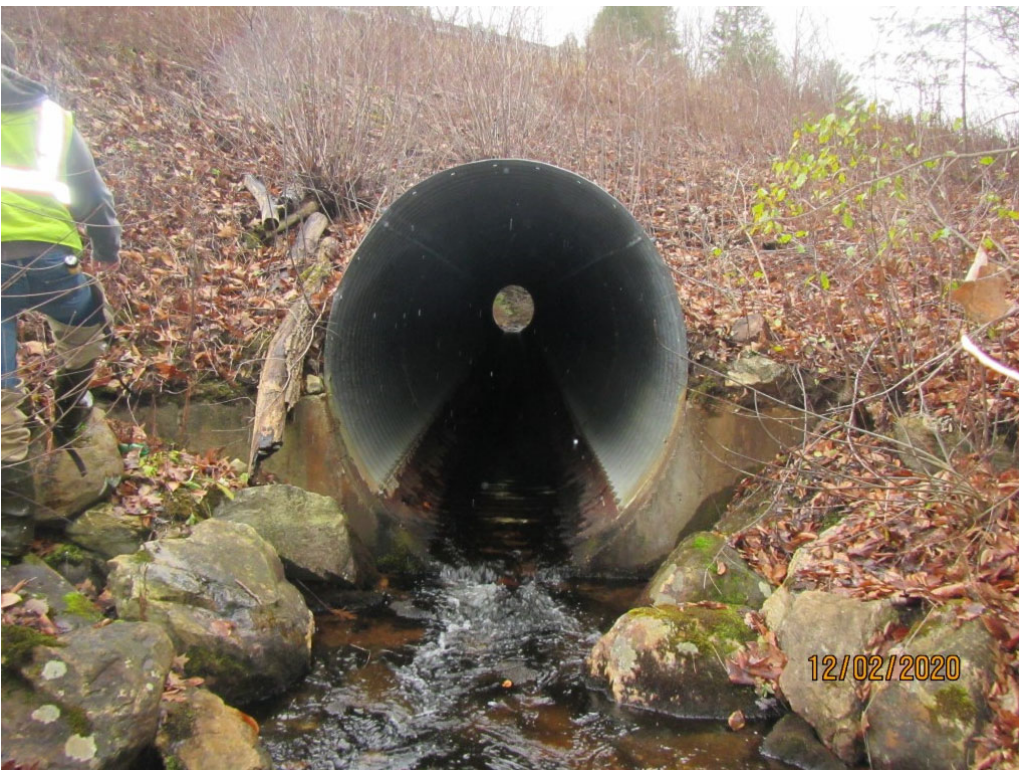
Picture 10: Culvert outlet
