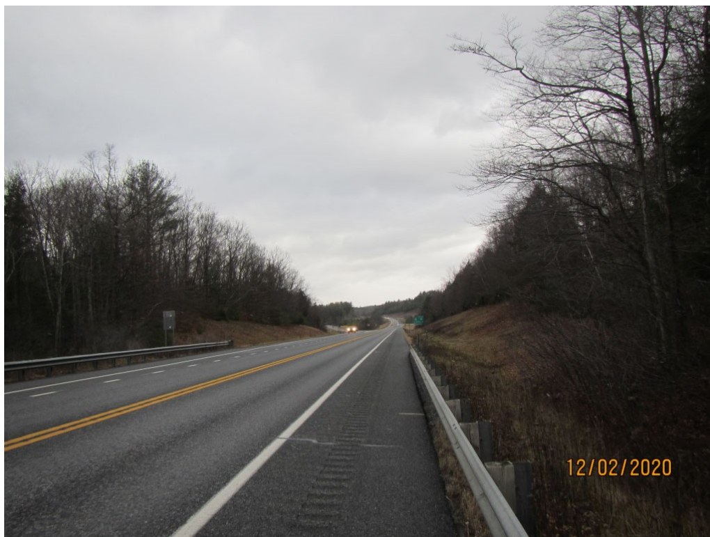
Picture 1: Looking north on US Route 7 over Bridge 19-7
